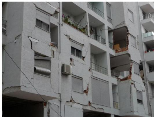
Figure 2. Earthquake-damaged infill walls, some of which have fallen out of the building.
