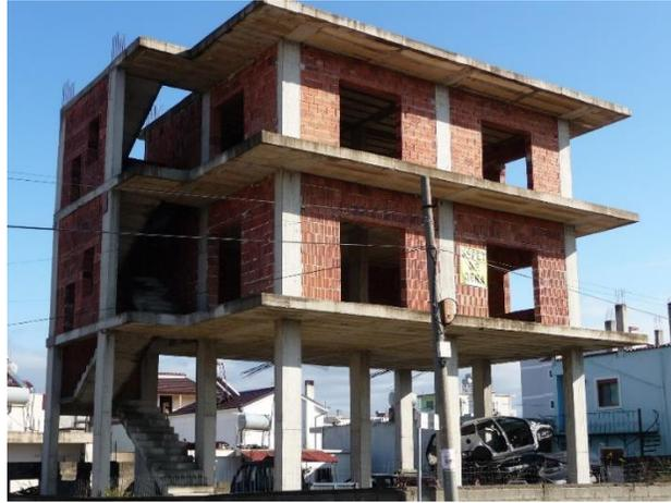
*Figure 5. A typical soft story building where the ground floor is the weakest.*
