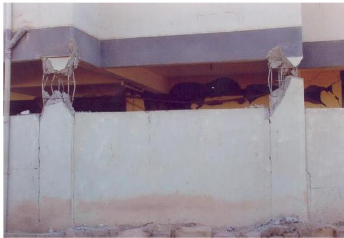
Figure 4. Earthquake-damaged short columns.
