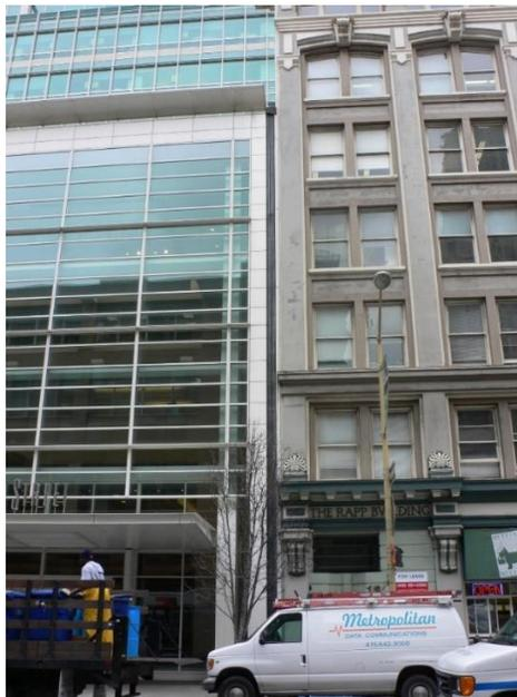
*Figure 4. Two buildings separated by a seismic gap covered by a flexible flashing.*
