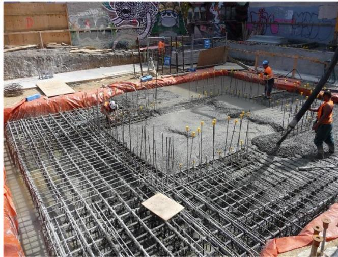
*Figure 3. The foundations of a building under construction. Engineers have followed codes to determine the amount of reinforcing steel and its correct location.*
