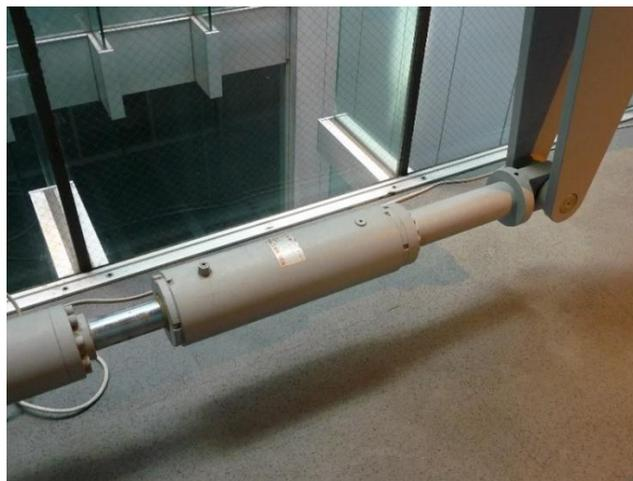
*Figure 3. A damper to reduce earthquake movements.*
