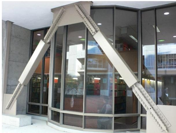
Figure 5. Two buckling-restrained braces resist and dampen down movement in an earthquake.
