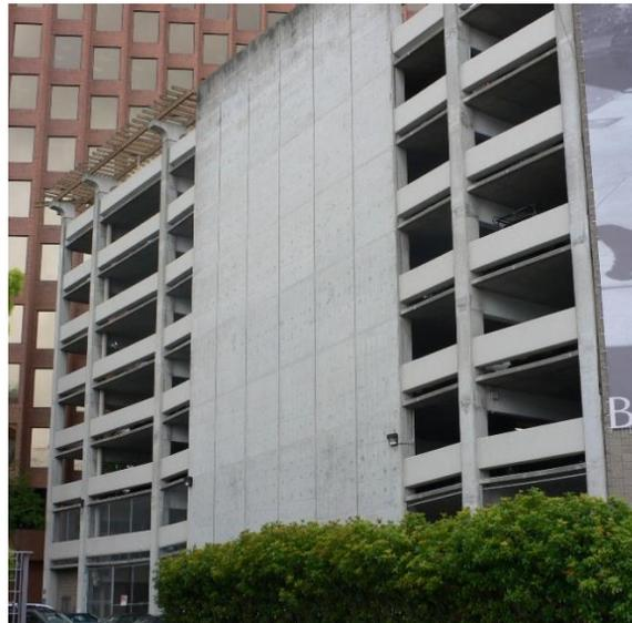
*Figure 4. A reinforced concrete structural wall resists forces acting along the length of the building. There should be another wall on the other side of the building.*
