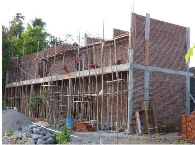
Figure 2. A confined masonry house under construction.
